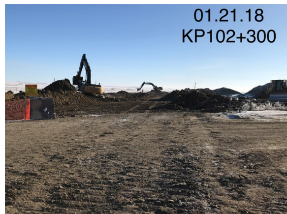
12. Excavators and dozers – Km 102+300 – Jan 21, 2018
