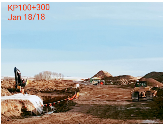
5. Dozer crossing – Km 100+300 – Jan 18, 2018
