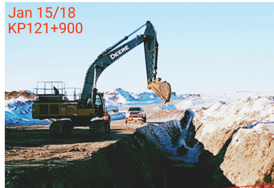
2. Excavator – Km 121+900 – Jan 15, 2018
