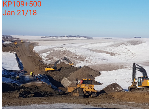
14. Backfill at ravine – 109km+500 – Jan 21, 2018
