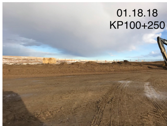
6. Excavator – km 100+250 – Jan 18, 2018
