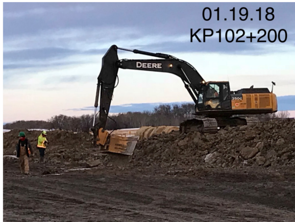
7. Excavator with sift bucket – Km 102+200 – Jan 19, 2018
