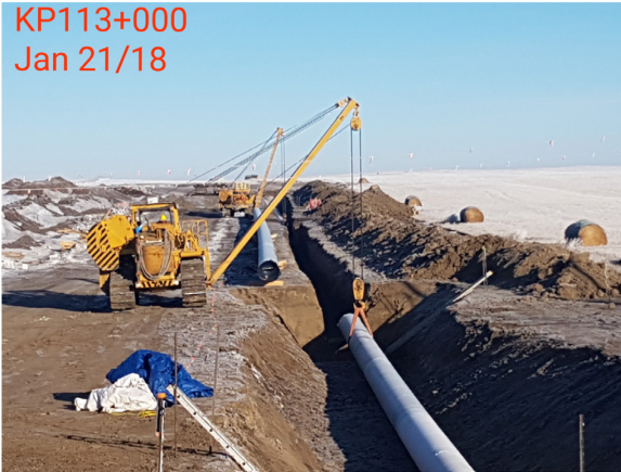
15. Tie-in welding – km113+000 – Jan21, 2018
