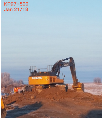
3. Bridge removal – Km 97+500 – Jan 21, 2018
