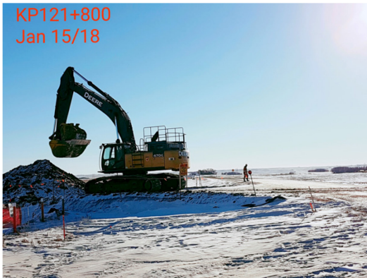
1. Excavator working on dirt piles- Km 121+800 – Jan 15, 2018
