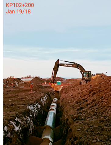
8. Excavator - Km 102+200 – Jan 19, 2018
